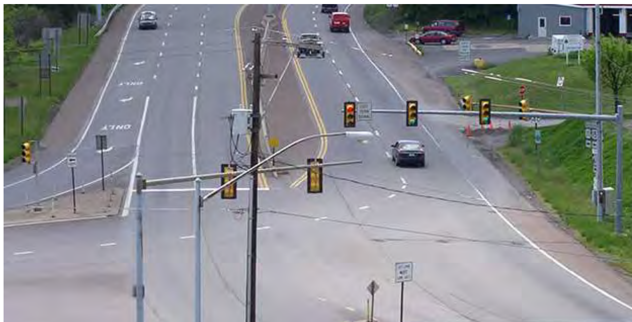
FIGURE 48: EXAMPLE OF A CONVENTIONAL TRAFFIC SIGNAL INTERSECTION
