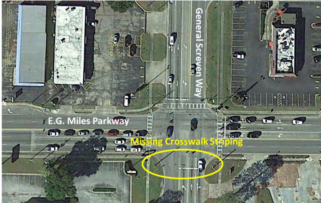
FIGURE 16: EXISTING MISSING PEDESTRIAN CROSSWALK AT E.G. MILES PARKWAY AND GENERAL SCREVEN WAY
