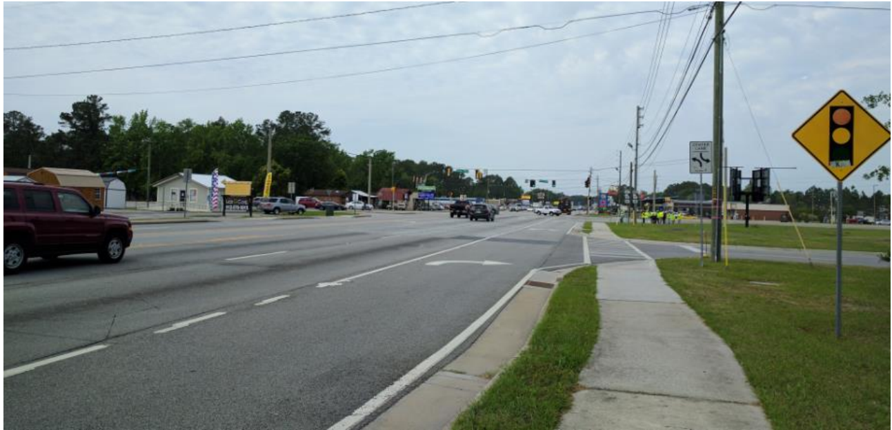
Figure 32: View of Westbound SR 196 at Veterans Parkway Intersection
